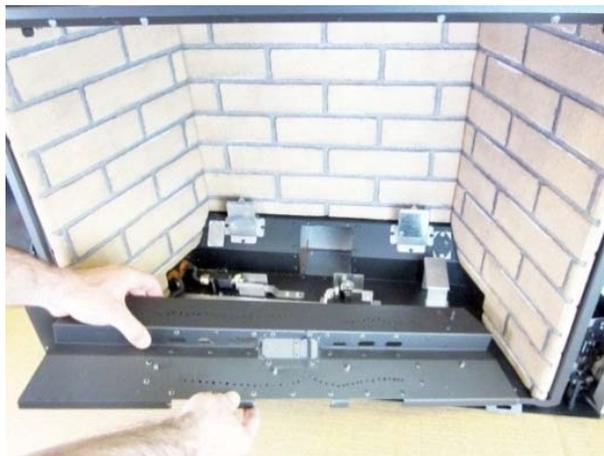
6. Replace the rear burner as shown.
