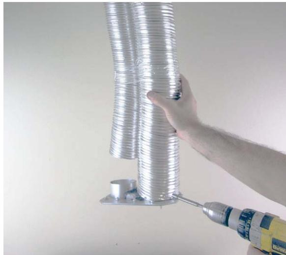
6. Attach the 3" intake vent to the connector and secure with at least 3 screws.
