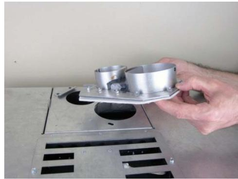
4. Make sure the gasket remains in place. Use silicone, if necessary, to secure the gasket.
