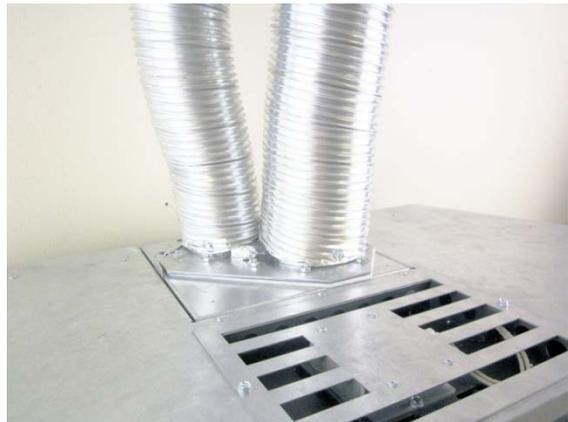
9. Re-attach the nuts removed in step 2 to secure the vent connector.
