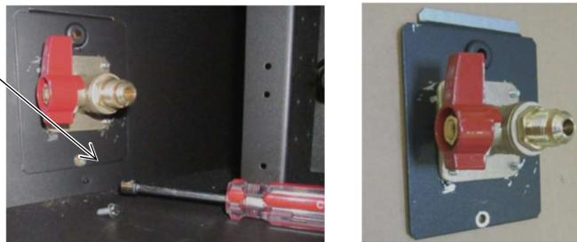
3. Remove the cover plate from the bottom of the fireplace (it is held in place in the same fashion as the shutoff valve plate). Attach it to the left side of the fireplace.
