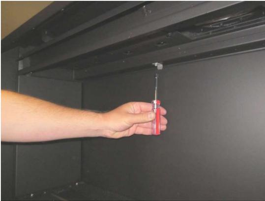
The fireback clip has a keyhole slot. It can be removed by loosening the screw and sliding the clip out.
