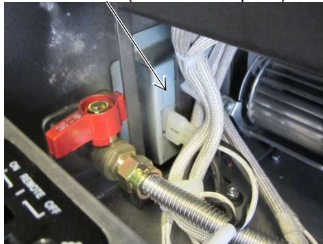
Junction Box (from inside fireplace)
