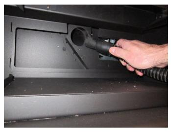
4. Clean the combustion blower with the bottle brush or vacuum.
