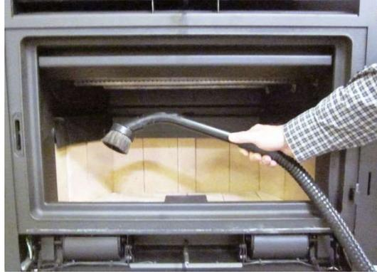
2. Carefully place the brush surface of the nozzle over the catalytic combustor openings and remove any ash or debris. Take care to prevent damage to the catalytic combustor (the surface is fragile).
