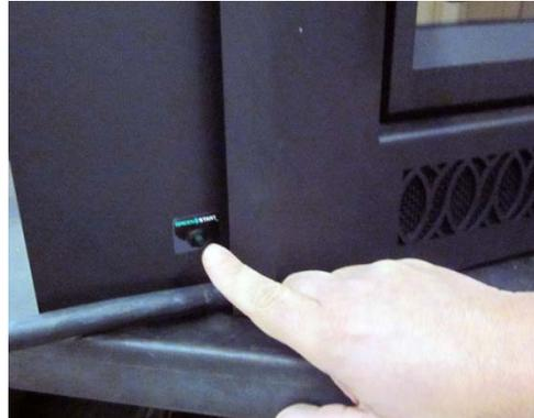
**NOTE:** If you need to turn off the igniter after starting the ignition process, press the GreenStart button a second time. The system will turn off power to the igniter and the GreenStart button will flash. The pump will continue to run for about seven minutes and then shut off.
