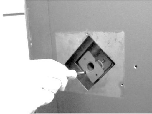
5. Attach the igniter with gasket to the igniter sleeve using the screws and gasket included in this kit. Note that the igniter gasket is placed between the sleeve and igniter assembly.
