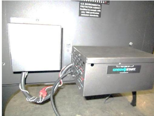
12. Plug in the compressor, then press the GreenStart start button.
