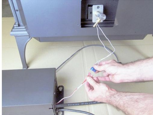
11. Attach the 1/4" tube to the nipple on the igniter.
