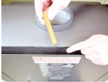
4. Remove the backing from the silicone gasket.
