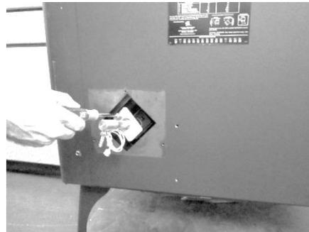
**NOTE:** These instructions show the compressor assembly attached to the back of the stove. Alternatively, you may place it on the floor near the stove. See the Cape Cod model installation instructions on page 12 for details.
